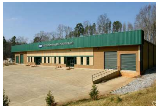
Our Distribution Center
